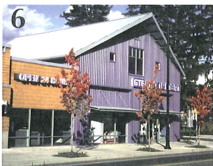
6 Storefront building with metal siding and pitched roof
