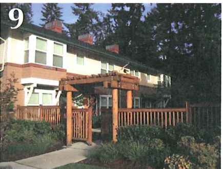
9 Multi-family building, 2-story
